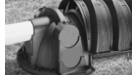
5. Insert inlet pipe.
