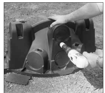
2. Drill hole with hole saw.
