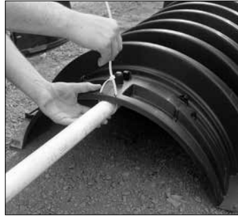
5. Secure the pressure lateral pipe.
