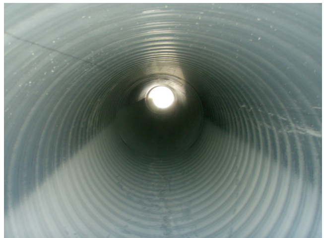
Smooth Interior Wall
