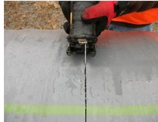
Figure 3: Incorrectly Cut Pipe
