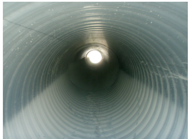
Smooth Interior Wall
