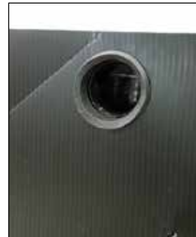
View from the outlet side
