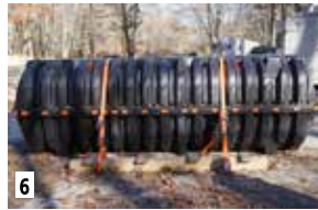
6 Position straps on tank.
