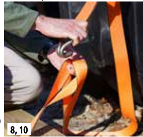
8, 10 Connect straps to beam.
