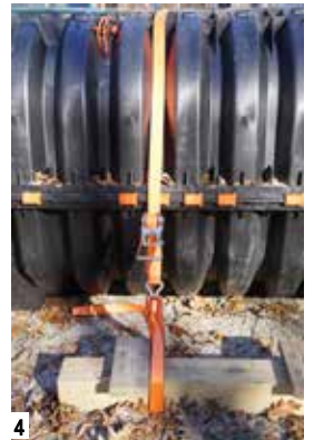
Position strap on beam.
