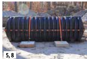
Position straps on tank.
