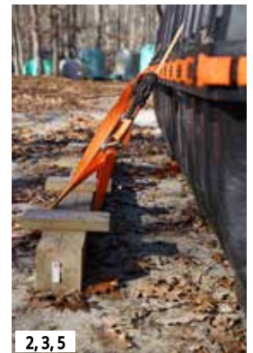
Position beam and tank.
