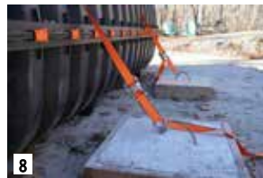
Connect strap to plate.
