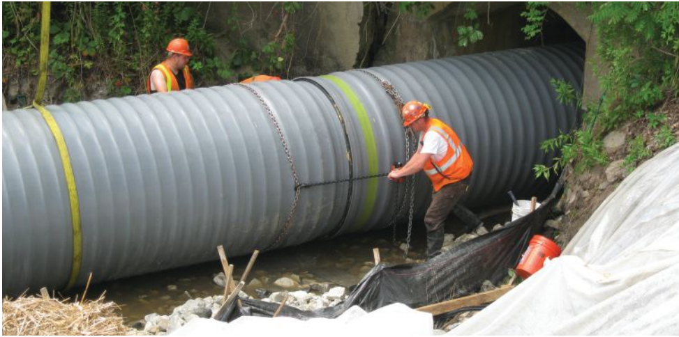
A contractor assembles the field joint with ratchet straps.
