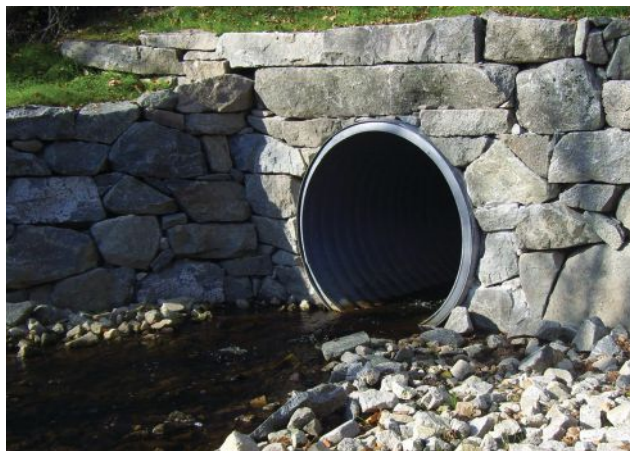
The final headwall and the 60-in.-diameter pipe blend in with the surrounding area.
