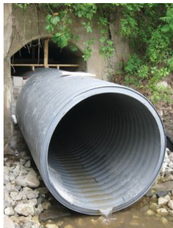
The final headwall and the 60-in.-diameter pipe blend in with the surrounding area.
