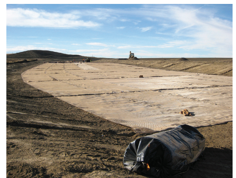
High-performance turf reinforcement mat with ultra-violet resistance for up to a 50-year design life in semi-arid conditions.
