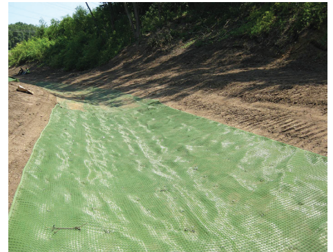
Woven turf reinforcement mat used for steep slope channel stabilization.
