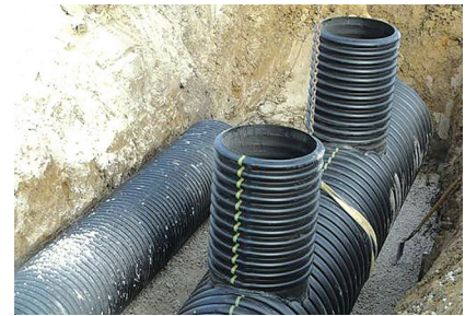
N-12 Water Harvesting Cistern
