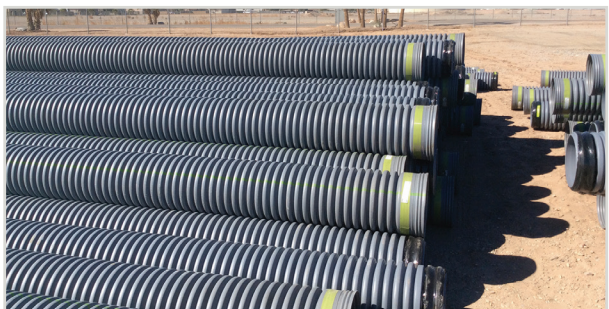
Stack pipe in a flat, clear area no higher than 1.8 m (6'). Use securing blocks to ensure pile does not collapse.
