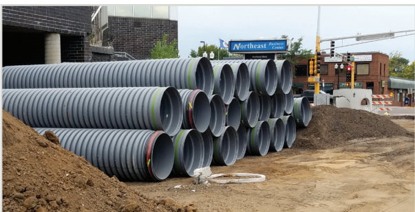
While supporting lengths of pipe evenly, alternate bells for each row of pipe.
