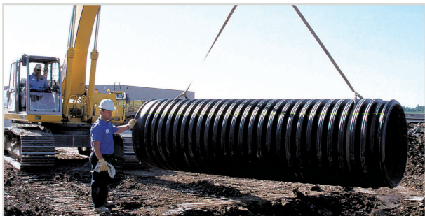
Lift 900 mm-1500 mm (36"-60") diameter pipe with sling at two points, spaced 3 m (10') apart.
