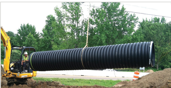
600 mm-750 mm (24"-30") diameter pipe requires a backhoe with one nylon sling.
