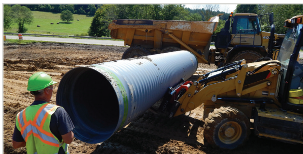
To prevent damage to the pipe, do not use forklift inside the pipe and avoid direct impacts. Do not drag or strike pipe ends against anything to avoid spigot or bell damage.
