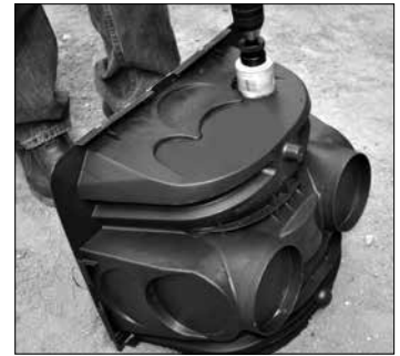
2. Drill pressure pipe hole.
