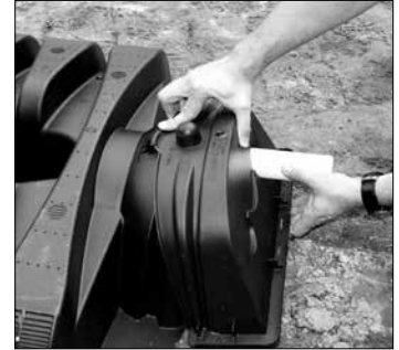
4. Place endcap over inlet end.
