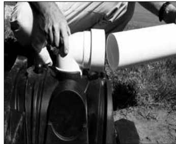
3. Connect inlet pipe.
