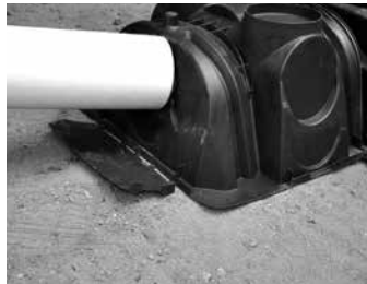
3. Insert inlet pipe.
