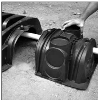
10. Lateral pipe through endcap.
