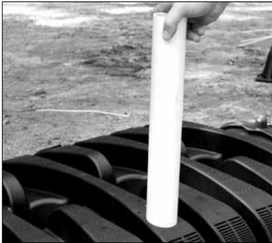
Chamber inspection port.
