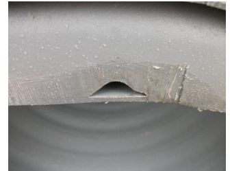
Figure 5: Drilling Vent Tube
