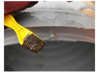
Figure 10: Finishing the Weld
