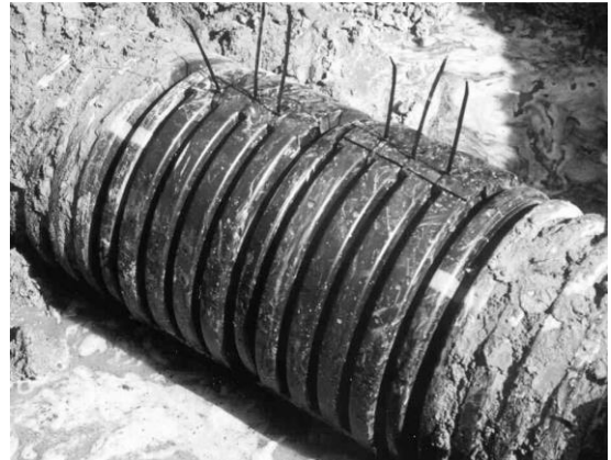
Figure 3 Split Band Installation
