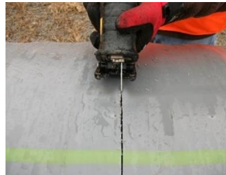
Figure 2: Cutting the Pipe
