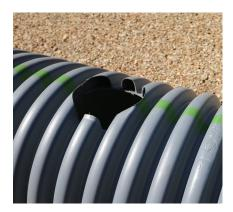
Core a hole perpendicular to the host pipe using the recommended hole saw. Remove the coupon from the saw. Deburr the cored hole.
