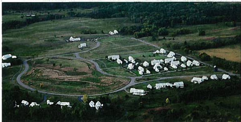
A 32-unit, private development in build-out mode in Marine on St. Croix, Minn., takes advantage of a decentralized wastewater treatment system designed by Natural Systems Utilities.
