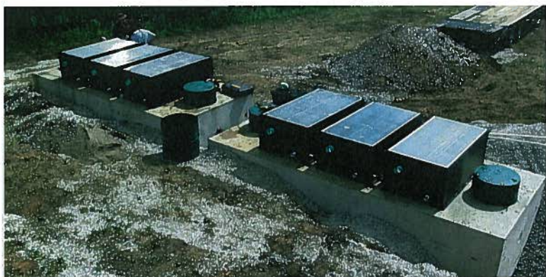
Oldcastle Precast's Bacpac Pretreatment System, shown here during construction, was installed at the OFS Cool Springs Corporate Education Center in Huntingburg, Ind.
