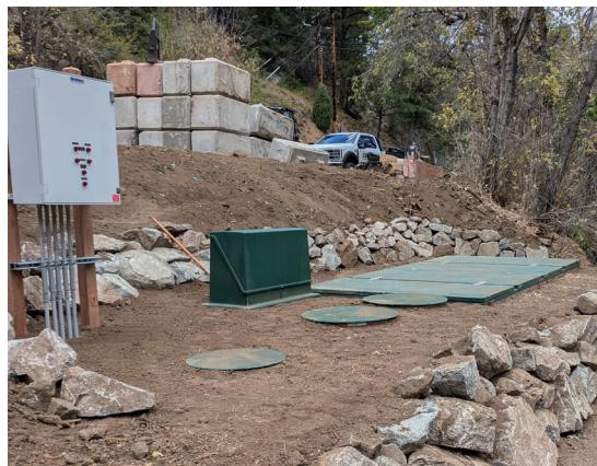
The installation included craning the septic tanks over the building to avoid shutting down the busy road. There was limited area for the tanks to be installed outside of the CDOT right of way. Access to import sand to the area was affected by the busy road and entrance on a curve. Due to limited access, CWS Excavating had to first install the water cistern tanks before the soil treatment area.
