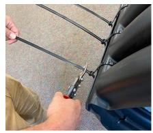
10. After the six zip ties have been zipped tight and ends have been trimmed, the split coupler has been installed.
