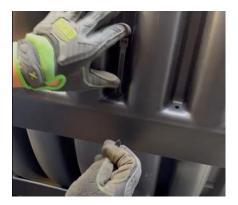
d. Complete securing the zip tie by feeding the pointed end of the tie into the square notch.
