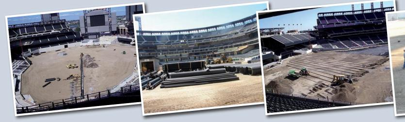
Underneath the field is a network of HDPE pipe that enables Bill Deacon, head groundskeeper, to create a vacuum to remove standing water or force cool or warm air into the root system of the natural grass.
