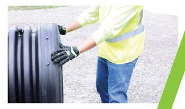
**STEP 4**: Check final location of gasket to make sure the gasket is properly positioned completely around the pipe.
