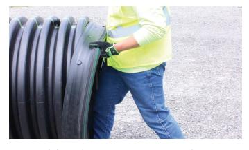
**STEP 2**: Slide gasket onto corrugation until it is difficult to stretch (typically ten and two o'clock positions).
