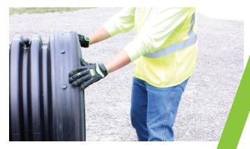
**STEP 4**: Check final location of gasket to make sure the gasket is properly positioned completely around the pipe. The green stripe should be positioned on the end of the pipe.
