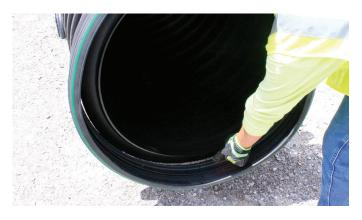
**STEP 1**: Initiate installation with gasket splice on bottom of pipe. NOTE: Gasket installation is more difficult in colder temperatures.
