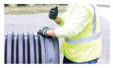
**STEP 3**: Use a pry bar to stretch the gasket into place. Use the exclusive pry hole technology built into the 24"-36" (600-900 mm) gasket. When gasket is in final location an audible "snap" will be heard.
