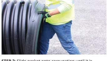
**STEP 2**: Slide gasket onto corrugation until it is difficult to stretch (typically ten and two o'clock positions).
