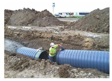
Lightweight and easily maneuverable ADS SaniTite HP polypropylene pipe helped increase efficiency in installing a new stormwater drainage line at Port Columbus International Airport.
