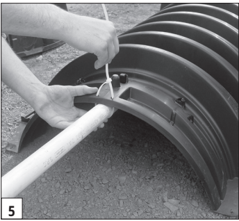
5 Secure with plastic strap.
