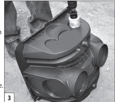
Drill pressure pipe hole.
