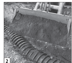
2 Backfill the soil.
