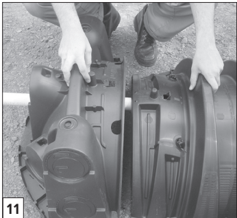
11 Insert pressure pipe.
