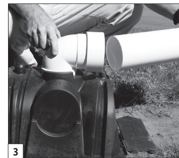
3 Connect inlet pipe
