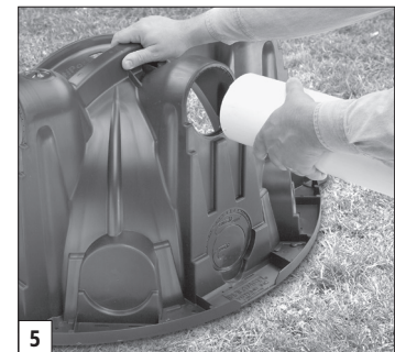
Insert inlet pipe.
