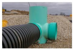
**STEP 3:** Install provided F-477 gasket for HDPE/PP corrugated pipe into last corrugation of the pipe. Lube the gasketed pipe and the inside of the drain basin bell.
