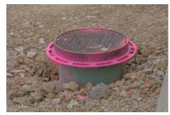
**NOTE:** For H-20 or heavier load rated installations, set elevation of frame and grate. Then pour a concrete collar around and knife flowable fill under edges to support the frame.
