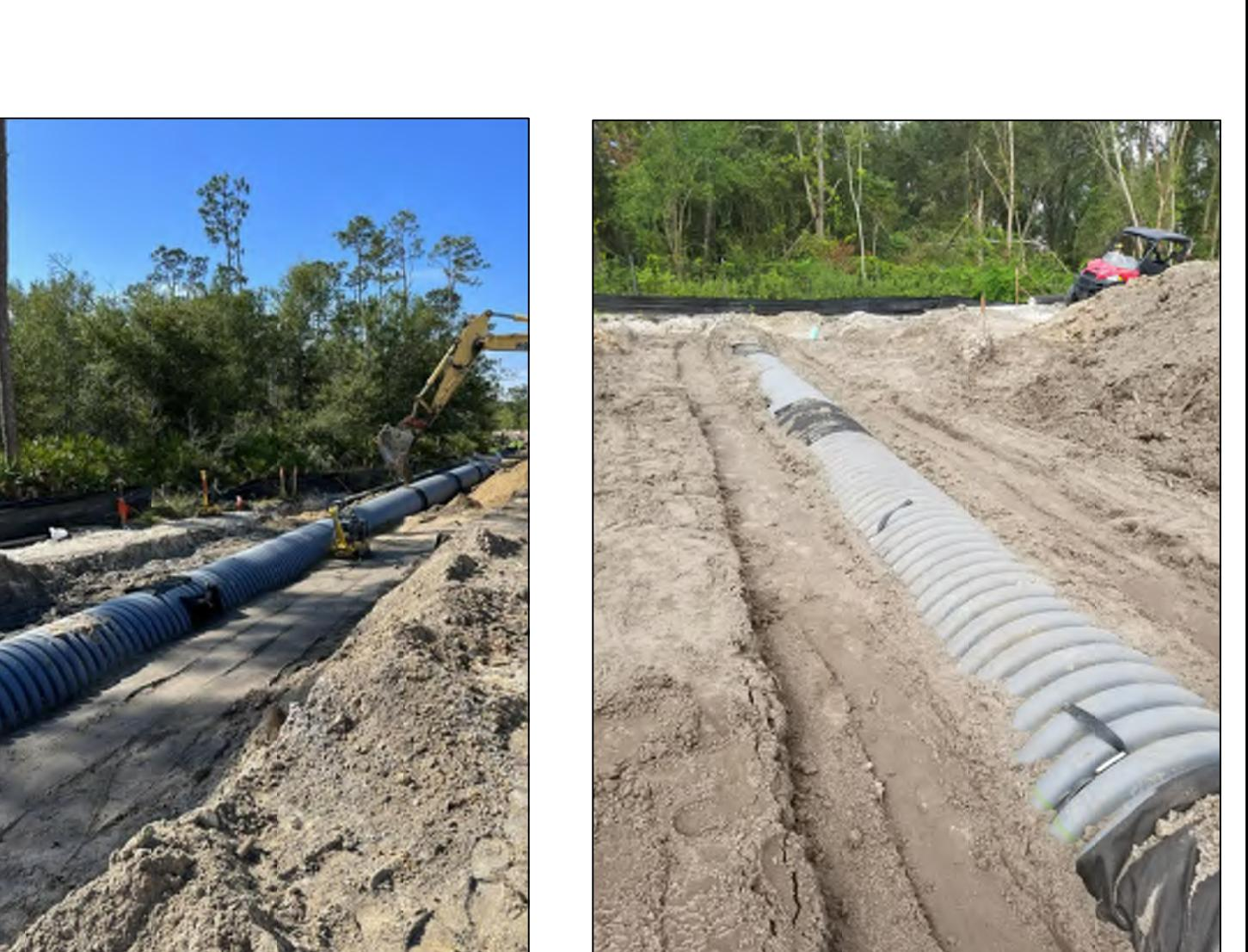
FOLLOW GUIDELINES SET FORTH IN SSBC SECTION 125. PLACE BACKFILL AROUND PIPE IN 6" COMPACTED LIFTS WITHIN PIPE COVER ZONE. COMPACT BEDDING AND BACKFILL WITH SMALL TO MEDIUM COMPACTION EQUIPMENT TO SPECIFIED DENSITY. VISUALLY INSPECT THE PIPE TO ENSURE THE APPROPRIATE SHAPE IS MAINTAINED.
