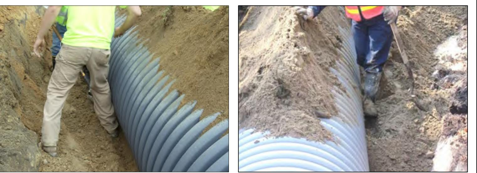
TRACKHOE OPERATOR SHALL UNIFORMLY PLACE A SHALLOW LIFT, OVER THE PIPE SO WORKERS CAN DIAGONALLY KNIFE OR BOOT PRESS SOIL UNDER PIPE HAUNCHES. PLACING BACKFILL UNDER THE PIPE HAUNCHES HELPS PREVENT THE PIPE FROM SHIFTING DURING BACKFILL COMPACTION.
