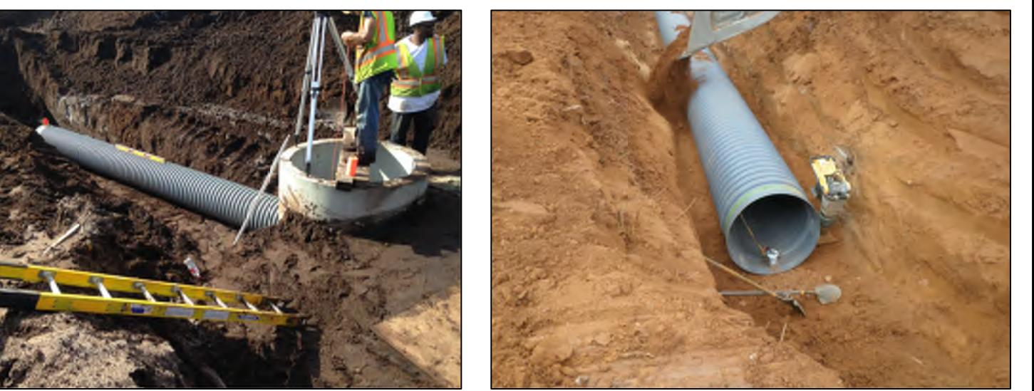
ENSURE BEDDING IS UNIFORM AND TRUE TO LINE AND GRADE. MIDDLE  $\frac{1}{3}$  SHOULD BE LOOSE TO CRADLE PIPE. CHECK 2-3 TIMES ALONG 20' STICK.
