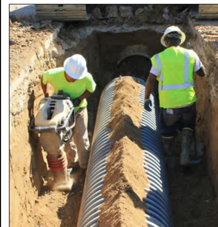
TRENCH MUST BE WIDE ENOUGH TO FIT PIPE, WORKERS, AND COMPACTION EQUIPMENT.
