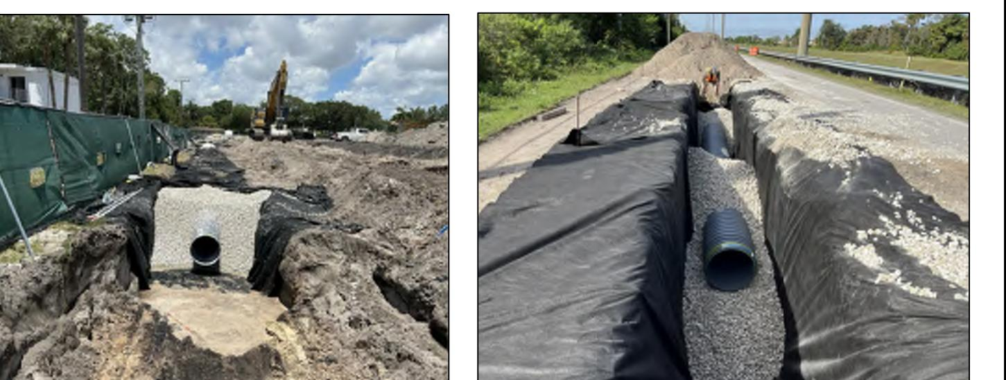
TRENCH SHOULD BE DRY OR PROPERLY DEWATERED BEFORE PLACING BEDDING AND BACKFILL. FOLLOW GUIDELINES IN 125-8.3.4 IF TRENCH IS UNABLE TO BE DEWATERED.
