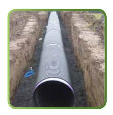
resin (PE 3408/PE3608) in the liner portion of the pipe. This resin is the same as that used in high pressure gas transmission lines throughout the United States. Although not required in traditional gravity-flow, non-pressure drainage applications, the addition of a pressure-rated resin allows continuous pressure (up to 5 psi) to be applied without detrimental long-term effects.
