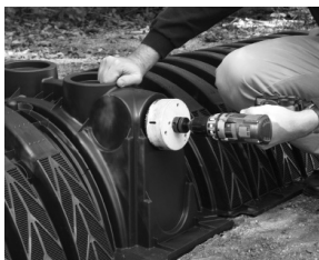
1. Drill endcap on side or top.
