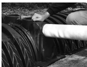
6. Insert connection pipe.
