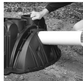
5. Insert inlet pipe.
