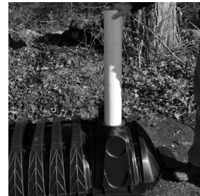
2. Pipe in endcap inspection port.
