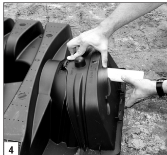
4 Place endcap over inlet end.
