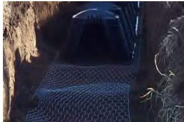
Figure 2: Install chambers over the wire
