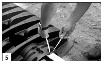
5 Secure pressure pipe.
