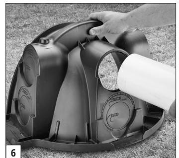
6 Insert inlet pipe.
