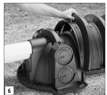
Place first chamber onto endcap.
