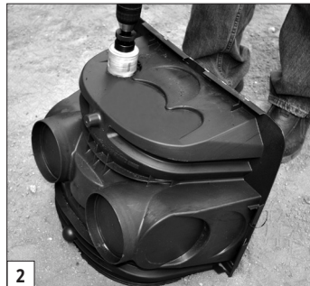
2 Drill pressure pipe hole.
