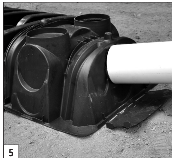
Insert inlet pipe.
