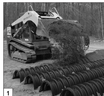
1 Ladle soil on chamber domes.
