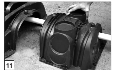
11 Lateral pipe through endcap.
