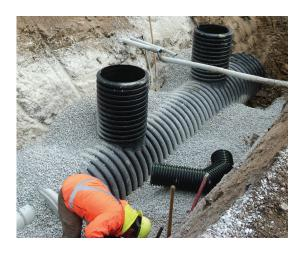
Installation of WQUs follows the same accepted practices as for the installation of large diameter flexible pipe. Specific installation instructions, along with details on specifying the proper size of a WQU, are available in Technical Note 1.03 and Installation Guide 2.01. You can also find more information on the ADS website *adspipe.com*.
