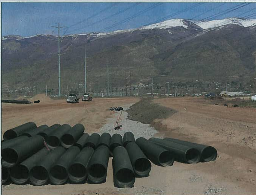
Here, the HDPE drainage pipe awaits installation, a process that is facilitated by its light weight requiring only one- or two-person crews.
