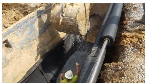
An initial layer of crushed stone bedding material was placed on top the geotextile, which was held in place on the side of the steel trench box with magnets.
