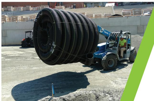
Networks of high-density polyethylene pipe would be needed. Rainwater would go into a pipe that also provides a way for the temperature controlled air to heat or cool the root zone. Another pipe would collect rainwater for field irrigation and another pipe system would be buried deeper to gather air for the geothermal system.
