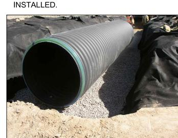
IF STONE OR ANY OPEN GRADED BEDDING MATERIAL IS USED, WRAP THE STONE WITH A MIN. 6 OUNCE NON-WOVEN GEOTEXTILE.
