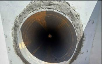
1) INSERT PIPE INTO STRUCTURE WITH PIPE RESTING ON BEDDING. THE PIPE SHOULD BE IN THE APPROXIMATE CENTER OF THE OPENING.
