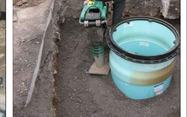
FINISHED GRADE PLACE BACKFILL IN 4"-6" COMPACTED LIFTS, TO **DENSITY REQUIRED AROUND PIPE IN TABLE 1** TAKE CARE TO ENSURE THE PIPE IS FULLY SUPPORTED BY BEDDING AND WELL
