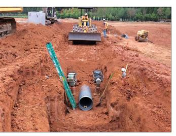
SEE TABLE 2 FOR MINIMUM COVER REQUIREMENTS FOR TYPICAL CONSTRUCTION EQUIPMENT.
