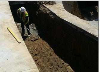
ENSURE BEDDING IS UNIFORM AND TRUE TO LINE AND GRADE. MIDDLE THIRD SHOULD BE LOOSE TO CRADLE PIPE
