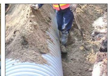
TRACKHOE OPERATOR SHALL UNIFORMLY PLACE A SHALLOW LIFT (NOT TO EXCEED 8"), OVER THE PIPE SO WORKERS CAN DIAGONALLY KNIFE OR BOOT PRESS SOIL UNDER PIPE HAUNCHES. PLACING BACKFILL UNDER THE PIPE HAUNCHES HELPS PREVENT THE PIPE FROM SHIFTING DURING BACKFILL COMPACTION. PLACE BACKFILL EVENLY ON BOTH SIDES OF THE PIPE TO PREVENT PIPE DISPLACEMENT, FOR ADDITIONAL GUIDANCE SEE ASTM
