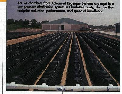
When compared with stoneand-pipe drainfields, chamber systems can accommodate a smaller footprint, yet their corrugated design provides up to 50 percent more infiltrative capacity and up to 67 percent more storage capacity, producers say.
