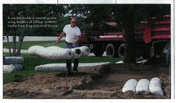
aquifer recharge areas, and in wellhead protection areas. The systems also retrofit into drainfields that have failed because of excessive organic loading.
