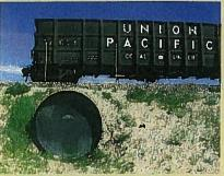
"The maximum measured combined deflection from construction and dynamic loading was less than 1.5 percent and the maximum deflection due to dynamic loads alone was 0.14 percent. The maximum measured tensile strains were negligible, and the maximum measured compressive strains were less than one percent. Operators noted that track ride quality was acceptable, and no track geometry maintenance was required at the conclusion of the test."
