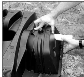
4. Place endcap over inlet end.
