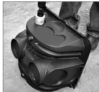
2. Drill pressure pipe hole.
