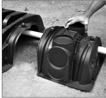
11. Lateral pipe through endcap.
