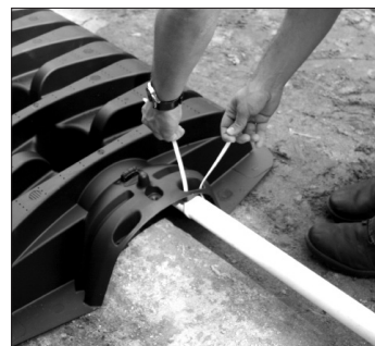
5. Secure pressure pipe.
