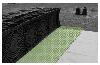
Install the next row of modules, over the geotextile. This row requires side panels be installed on the module sides facing the Isolator Row.
