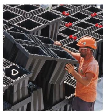
The Aquabox Cube has a central opening which enables a 12" (300 mm) N-12 riser pipe to reach the surface. A Nyloplast inline drain finishes the top of the riser pipe.
