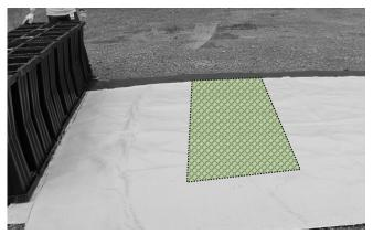
Begin with one layer of ADS Plus geotextile below where the Isolator Row will be installed. After installing the modules two rows away from the Isolator Row, roll out a second layer of ADS Plus abutting the modules.
