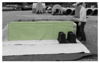
Once the the Isolator Row modules are installed, fold the upper layer of ADS Plus geotextile back over the top of the Isolator Row. Begin installing the next row of modules to hold the geotextile in place.
