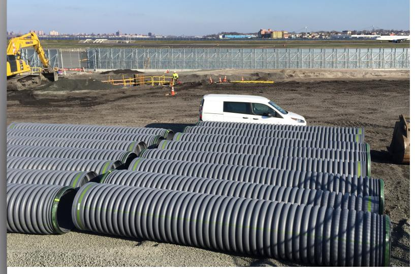
More than 50,000 feet of thermoplastic stormwater drainage pipe is being used to construct the new system at LaGuardia Airport in New York City.
