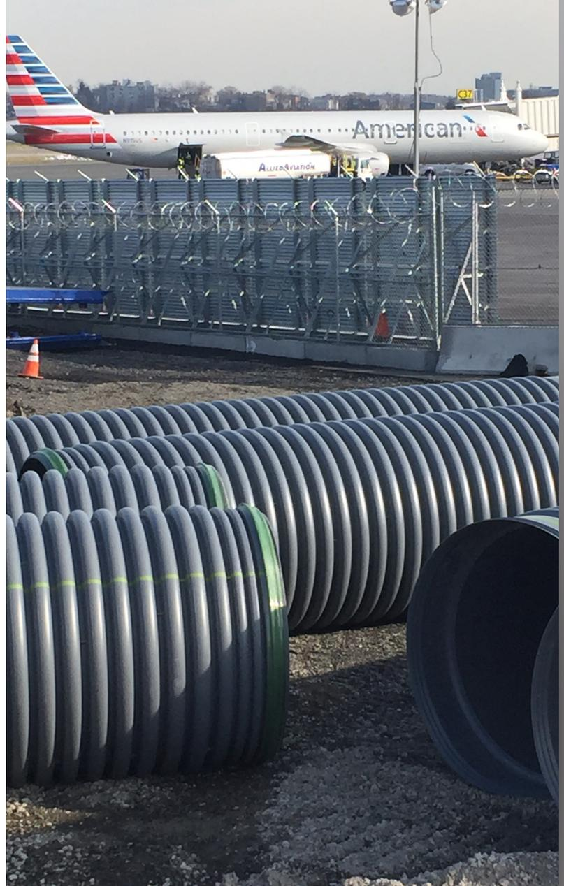
Use of ADS N-12 HDPE and HP Storm pipe allowed for faster installation and improved joint performance. This provided the contractor with flexibility in coordinating the drainage installation with other portions of the project that have less flexible schedules, which reduced installation costs while providing an improved drainage system with a life expectancy of more than 75 years.
