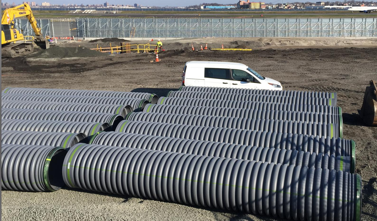
More than 50,000 feet of thermoplastic stormwater drainage pipe is being used to construct the new system at LaGuardia Airport in New York City.
