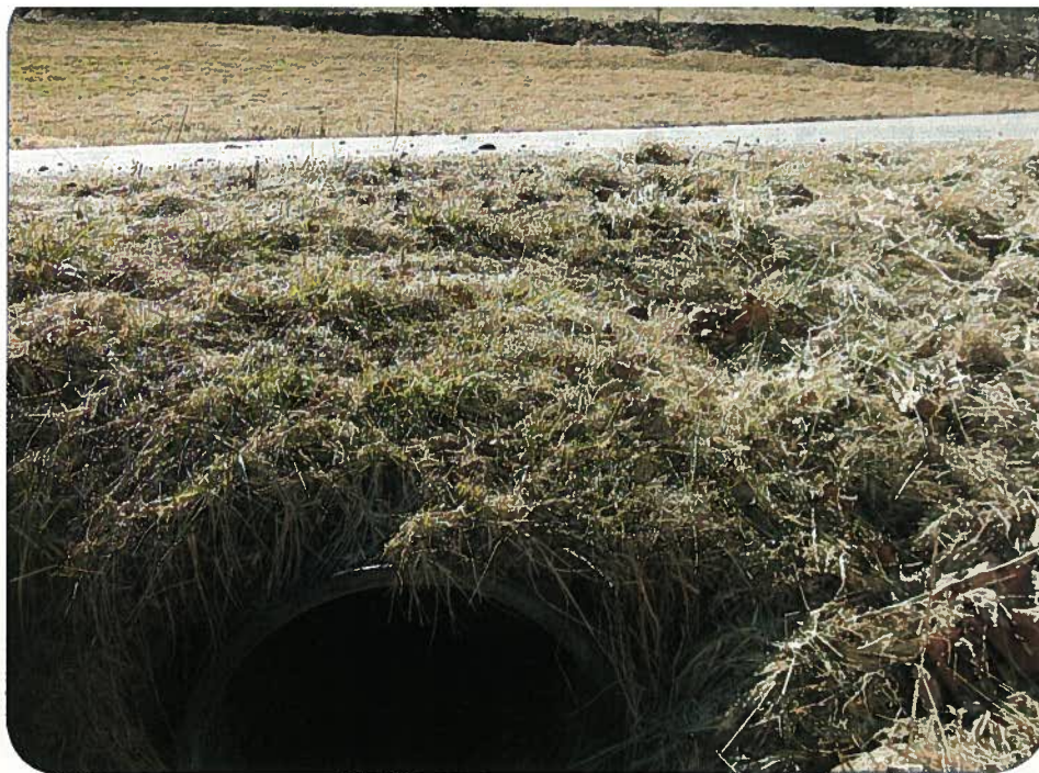
The HDPE pipe runs under Rte. 145 and collects acidic runoff from abandoned strip mines.
