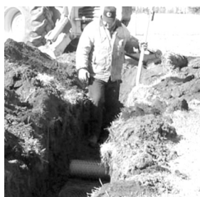
Figure 1: Roll out chicken wire on trench bottom
