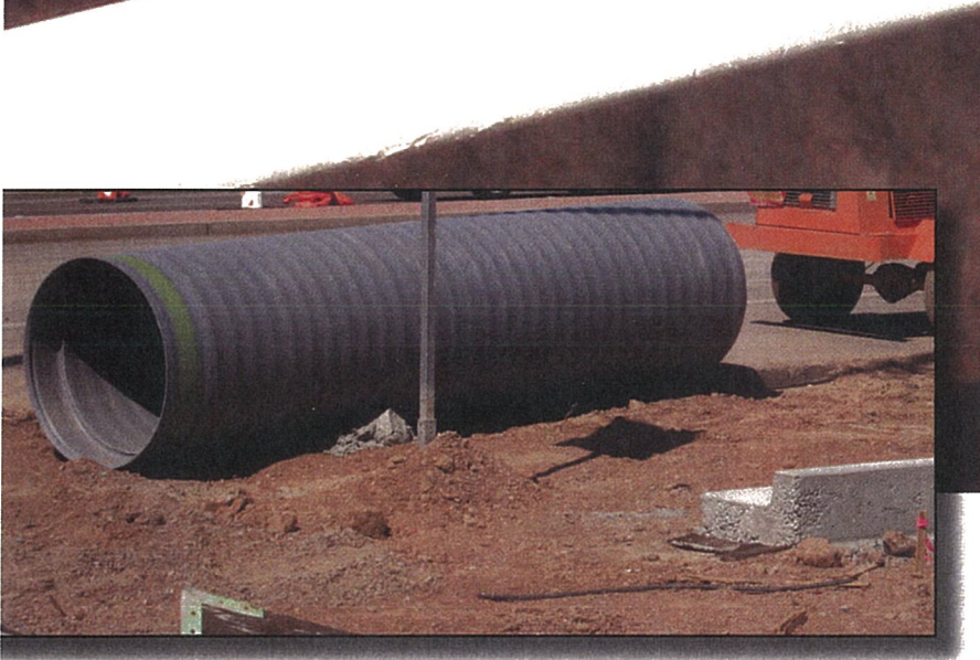
pipe is made from an engineered grade of polypropylene resin.
