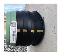
Inner sleeve may not go all the way through the concrete, but it does not have to. It will seal to concrete and stay in place.
