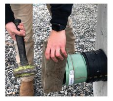
Drive the plastic hub into the rubber sleeves with a 4 pound mallet and block of wood. Stop when the rubber sleeve meets the red line.
