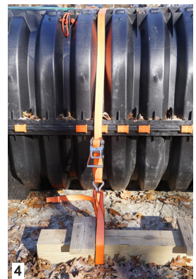
Position strap on beam.
