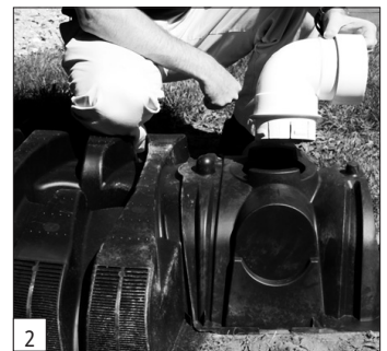
Insert Quick4 Plus Periscope.
