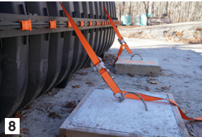
Connect strap to plate.
