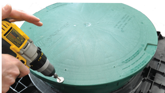
Prior to backfilling, fasten the lid to the riser with screws provided.
