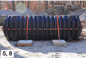
Position straps on tank.
