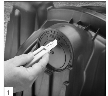
Start tear-out seal.
