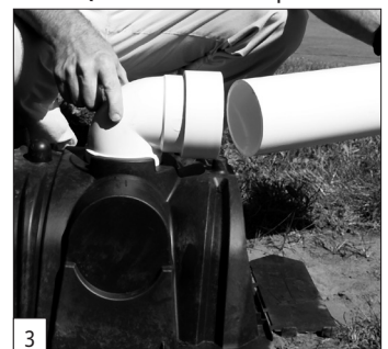
Connect inlet pipe.
