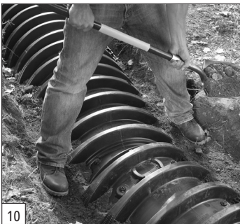
Attach endcap to last chamber.
