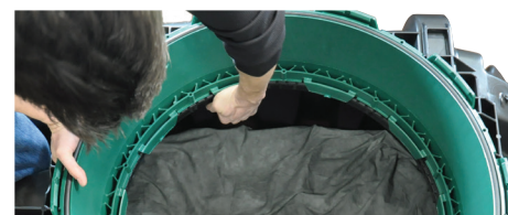
Engage one set of tabs into proper position.
