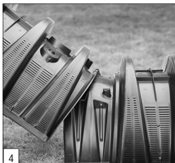
Place first chamber onto endcap.
