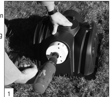
Drill endcap on side or top.
