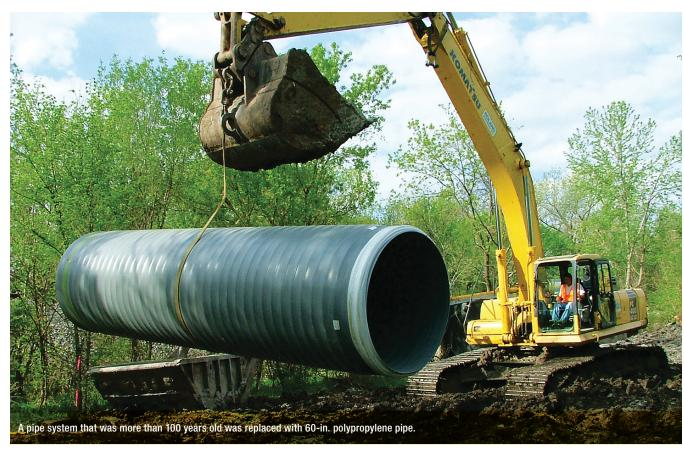
connect to the Taylor Street CSO as a way to reduce inflow and infiltration by replacing the old brick sewer with a larger diameter pipe, as well as eliminate a bottleneck under Morley Street.
