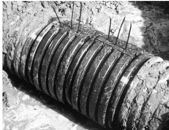
Figure 3: Split Band Installation
