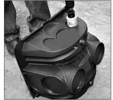
2. Drill pressure pipe hole.
