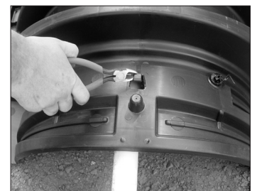
9. Remove the tongue if necessary.
