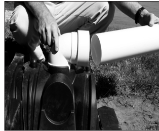
3. Connect inlet pipe.
