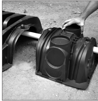
10. Lateral pipe through endcap.
