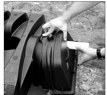
4. Place endcap over inlet end.
