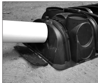
3. Insert inlet pipe.
