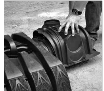
4. Place endcap over inlet end.
