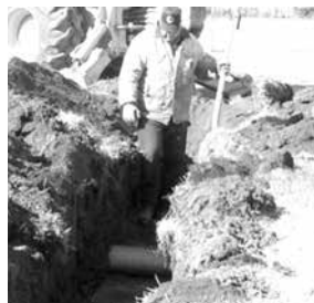
Figure 1: Roll out chicken wire on trench bottom
