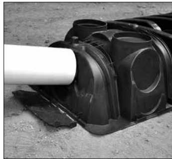
5. Insert inlet pipe.
