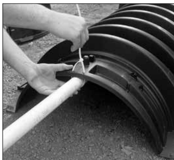
5. Secure the pressure lateral pipe.
