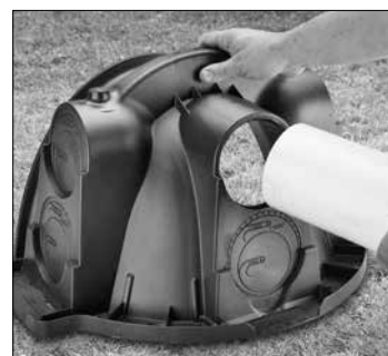
5. Insert inlet pipe.
