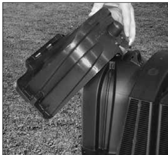
1. Attach endcap to last chamber.
