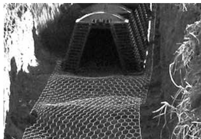
Figure 2: Install chambers over the wire base
