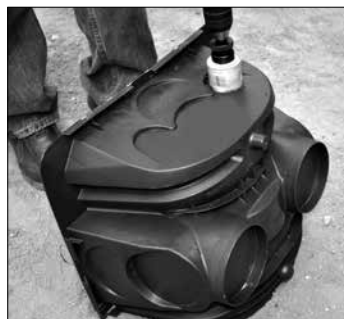
3. Drill pressure pipe hole.
