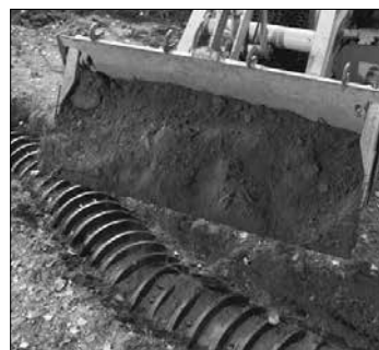
2. Backfill the soil.
