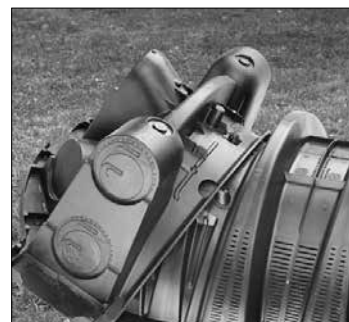
6. Attach endcap to chamber.
