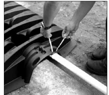
5. Secure pressure pipe.
