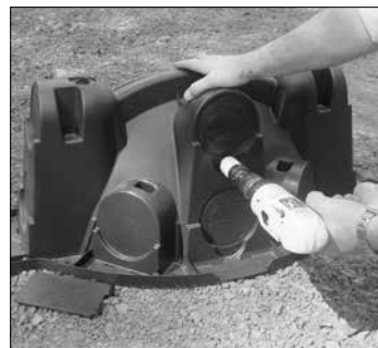
2. Drill hole with hole saw.
