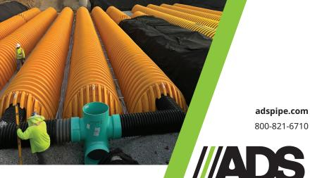
Kimley-Horn knew that StormTech MC-7200 Stormwater Chambers would be the ideal detention system, while HP Storm pipe could convey stormwater to the chambers. Existing Nyloplast basins in the park were used to capture the stormwater. The engineering firm had previously utilized ADS products and knew the cost effectiveness, versatility, ease of installation and maintenance would save the city money.
