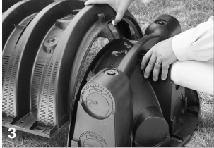
3 Place first chamber onto endcap.
