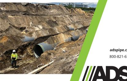
adspipe.com 800-821-6710 Smaller diameters of HP Storm, from 24"-36" (600-900 mm), were also used to convey stormwater to the double barrel run. An 80' (24 m) run of 48" (1200 mm) HP Storm was utilized to fill an open water ditch. Closing the ditch moved all the stormwater underground to avoid open water and to keep birds away from the runway to help prevent bird strikes.
